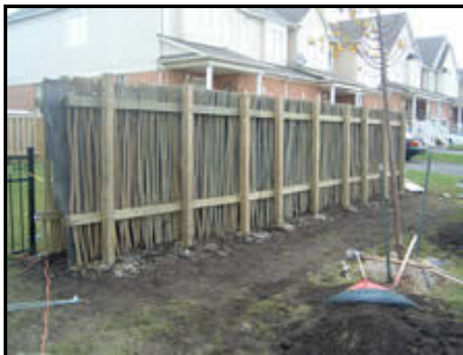
The Living Wall, after installation
