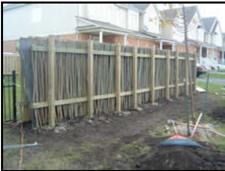
The Living Wall, after installation
